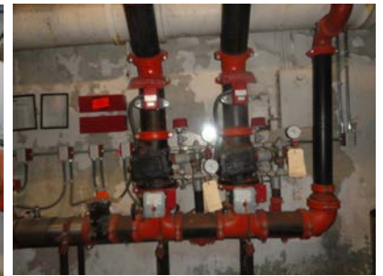
Photo 3: Existing Fire Protection Risers
