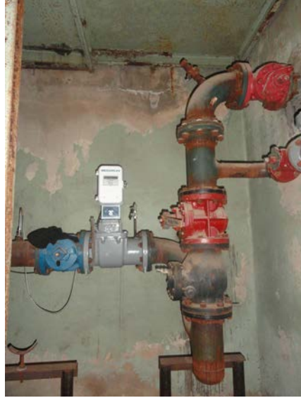
Photo 7: Existing 10 inch Gas Piping
