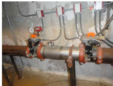
Photo 2: Existing Double Check Valve Assembly
