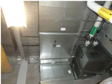
Photo 6: Fixed Obstructions Over 4 Feet Wide that are not Protected in the New Building
