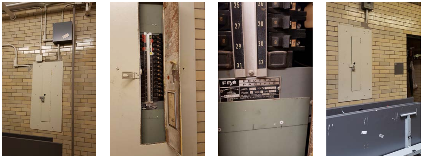
Photo 4: Examples of Old Panelboards
