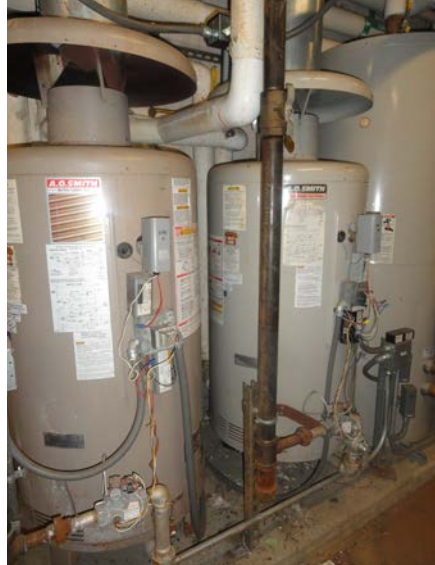
Photo 3: Existing Water Heaters, Storage Tanks and Thermal Expansion Tank
