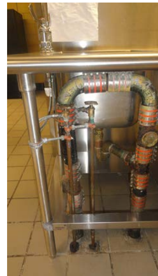
Photo 14: Bow Venting at Island Sink
