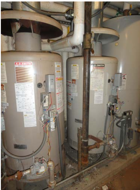
Flues Disconnected from Domestic Water Heaters Venting
