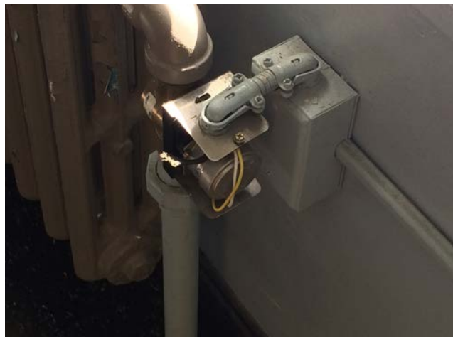
Original Pneumatic Control Valve
