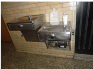
Photo 20: Existing Bi-Level Electric Water Cooler (EWE)
