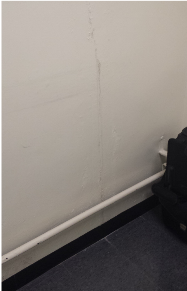
Crack in Wall Finish
