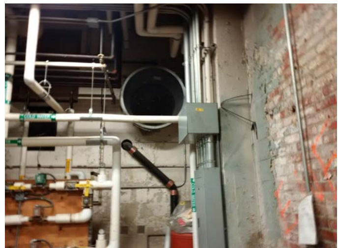
Boiler Room Open End Ventilation/Combustion Air Duct
