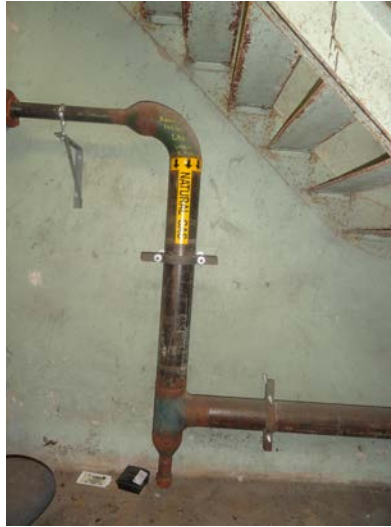
Photo 9: Existing 5 inch Gas Piping
