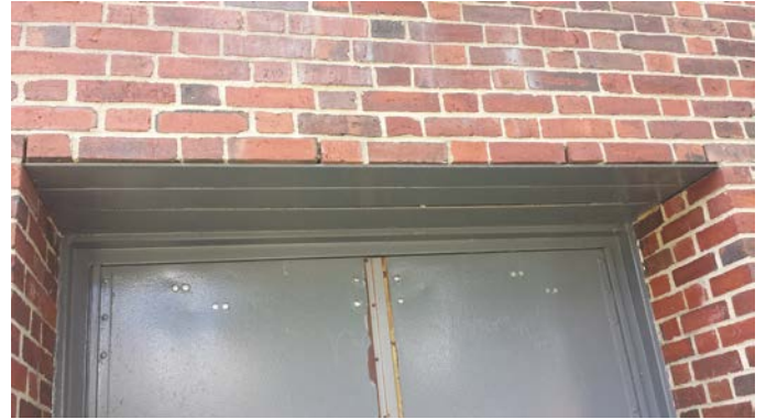
Cleaned and Repainted Lintel
