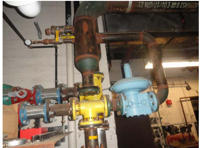
Photo 7: Existing 10 inch Gas Piping
