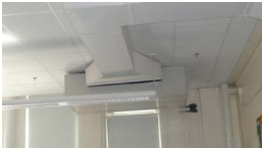
Photo 5: Examples of Sprinklers that are obstructed by HVAC Unit/Duct in the Original Building
