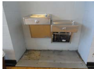
Photo 20: Existing Bi-Level Electric Water Cooler (EWE)
