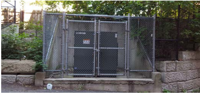
Photo 1: Pad-Mounted Transformer
