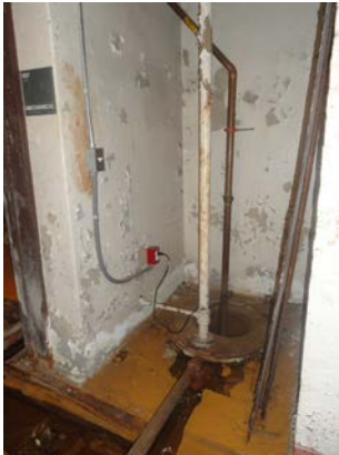
Photo 10: Existing Sump Pump
