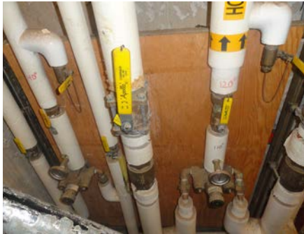
Photo 4: Existing Domestic Water Piping and Mixing Valves
