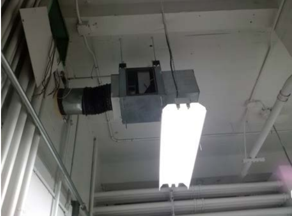
Electrical Room Exhaust Fan with Disconnected Wiring
