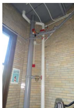
Photo 4: Floor Control Valve Assemblies in the Original and New Buildings
