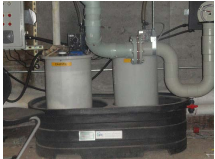
Photo 15: pH Adjustment System
