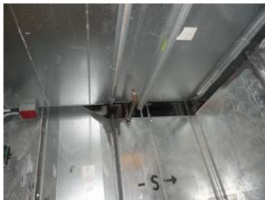
Photo 7: Examples of Sprinklers Installed Below HVAC Unit/Duct that do not have Guards in the New Building
