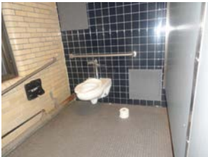
Photo 19: Existing Plumbing Fixtures; Non-ADA Compliant
