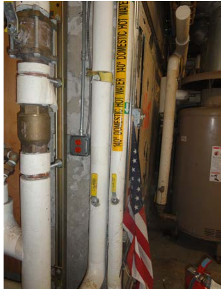
Photo 5: Existing Domestic Hot Water Circulation Piping and Pumps
