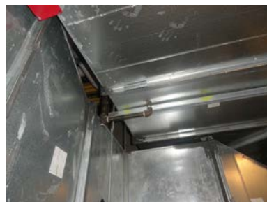
Photo 7: Examples of Sprinklers Installed Below HVAC Unit/Duct that do not have Guards in the New Building
