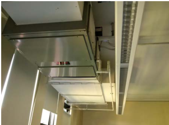
Air Conditioning Condensate Drain Piped Directly through window to discharge outside
