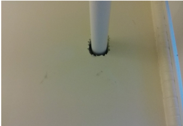
Missing Seal around at Piping Wall Penetration
