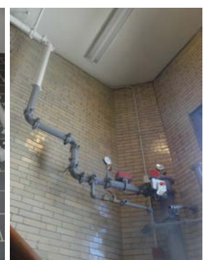
Photo 4: Floor Control Valve Assemblies in the Original and New Buildings
