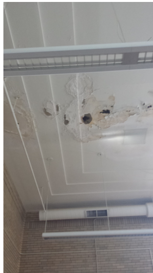
Ceiling with Water Damage from Roof Leaks
