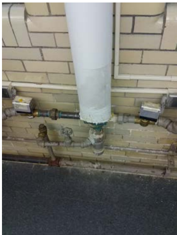
Retrofitted Control Valves
