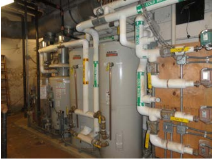
Photo 3: Existing Water Heaters, Storage Tanks and Thermal Expansion Tank
