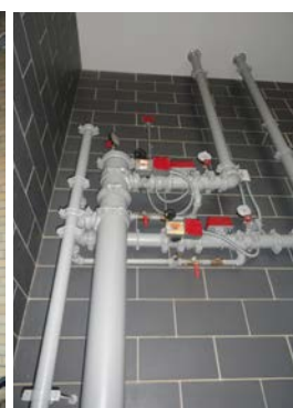
Photo 4: Floor Control Valve Assemblies in the Original and New Buildings
