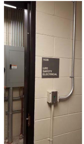
Photo 6: Example of "Emergency Power" Closet
