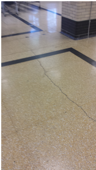
Crack in Terrazzo at Tunnel Slab
