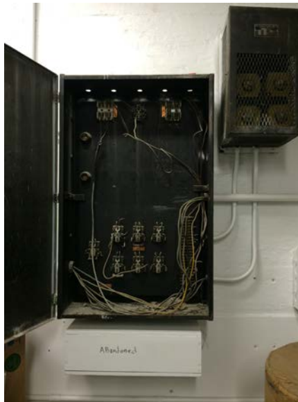
Abandoned Systems in Main Electric Room
