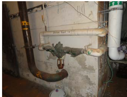
Photo 2: Existing Backflow Preventers for HVAC Make-up
