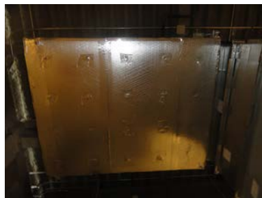
Photo 6: Fixed Obstructions Over 4 Feet Wide that are not Protected in the New Building
