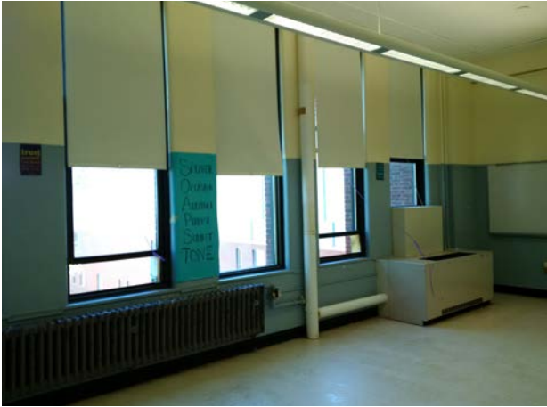
Classroom Unit Ventilator and Finned Tube Radiation
