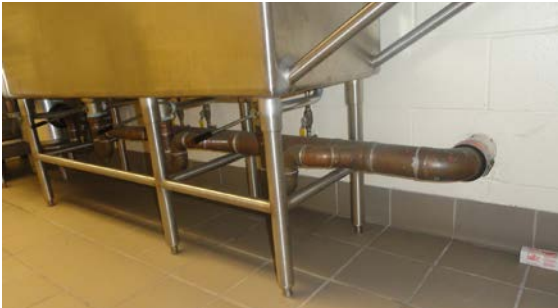
Photo 12: Piping Installation at Triple Pot Sink
