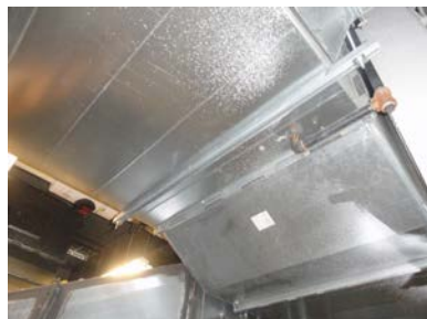
Photo 7: Examples of Sprinklers Installed Below HVAC Unit/Duct that do not have Guards in the New Building
