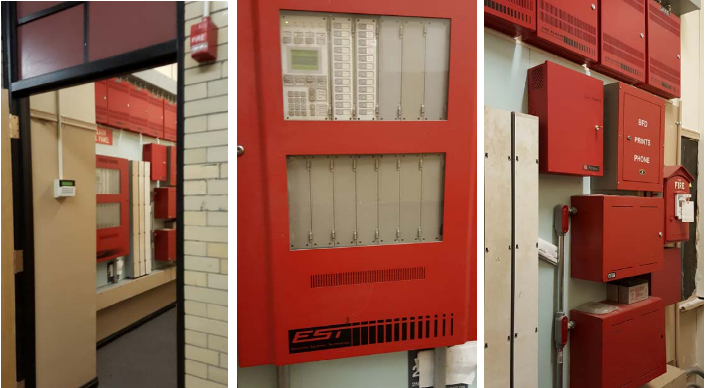
Photo 9: Existing FACP and Associated Equipment
